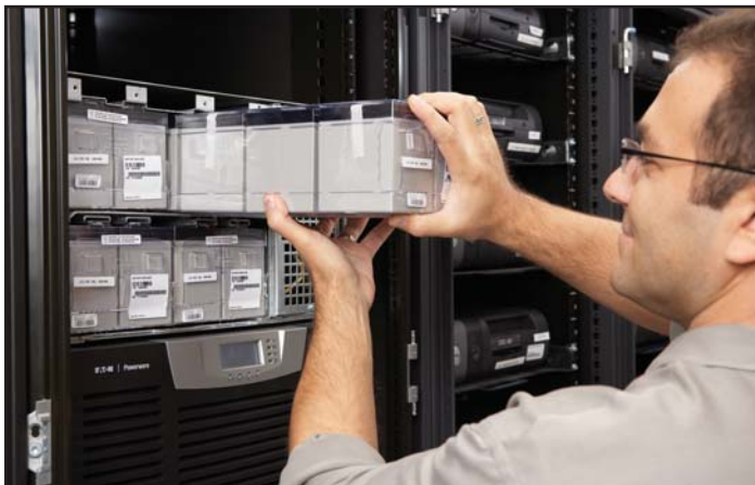
IT staff can easily replace battery modules.
